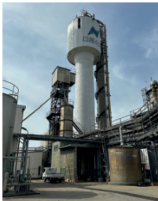
Granulation Tower: Symbol of Toiyama Plant
